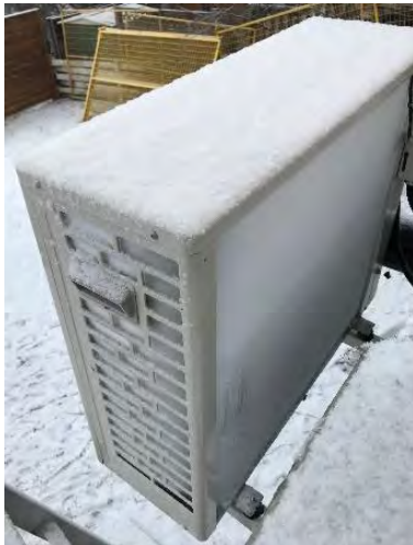
Figure 49: The Eco2 heat pump water heater compressor working outside in 5°F (-15°C) weather. 104
