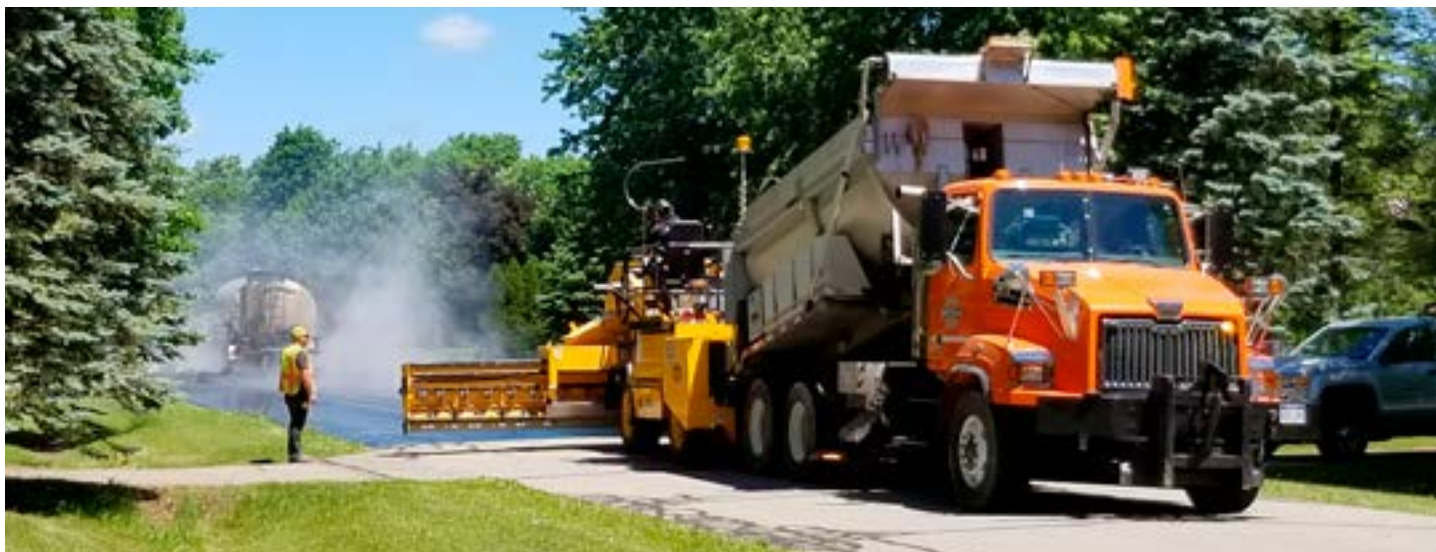
Local road being sealcoated through the township's special assessment district local roads program.
