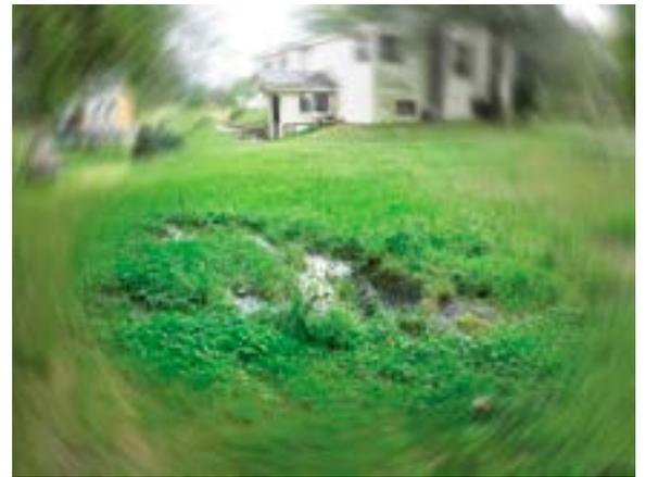
*This water on the lawn tells a tale: it's time to fix the septic system. The average cost of replacing a septic system is \$9,000-\$15,000. Regular inspections and maintenance will save money in the long run.*
